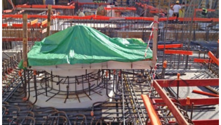
JHR vertical docking port for transport casks, part installed on site
